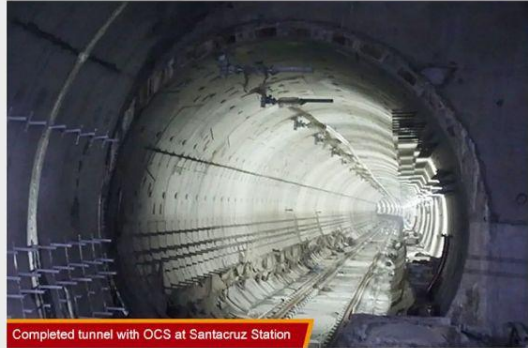
Completed tunnel with OCS at Santacruz Station
